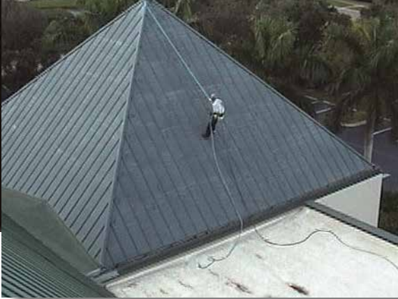
Naples Philharmonic, Naples, Florida (In-progress view)
