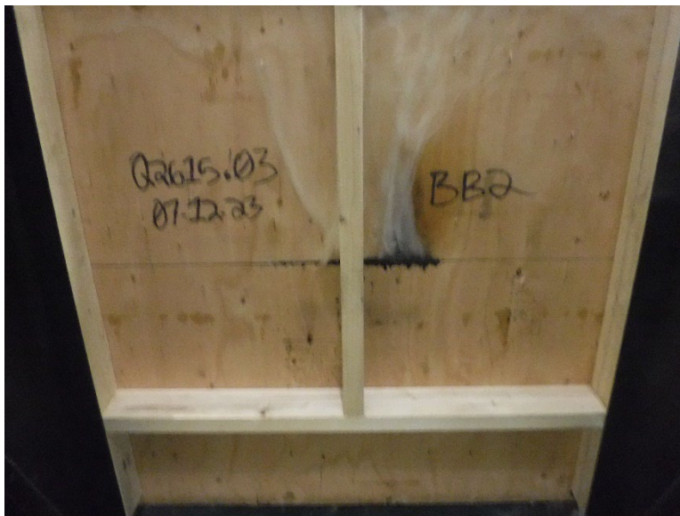
Photo No. 10 TEST #2 Underdeck During Test
