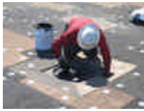
Performing detail work on the drain
