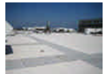
The finished roof system
