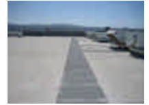
The finished roof system
