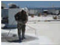
Spray application of the adhesive
