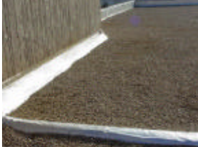
American Electric Power Buchanan, Michigan
