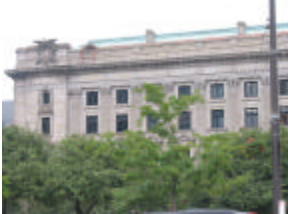
Metzenbaum Federal Courthouse Cleveland, Ohio
