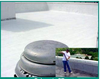
Polarcote FR Energy Star certified Acrylic latex roof coating used as a final surface coat over smooth asphalt emulsions, flashings and modified bitumen membranes Reflects solar radiation to lower surface temperature and slow the roof aging process Can help reduce energy costs Increases a roof's fire resistance and rating Excellent waterproofing characteristics
