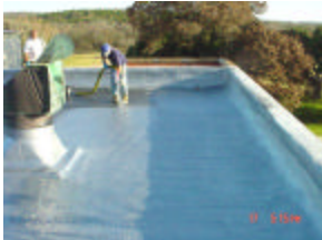
Reflective Coating, Veteran's Administration Medical Center, Kerrville, TX
