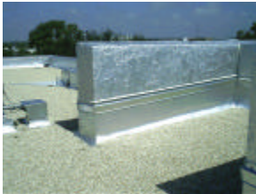
Hypalon Flashing Detail and Wall Coating Frio County Courthouse Frio County, Texas
