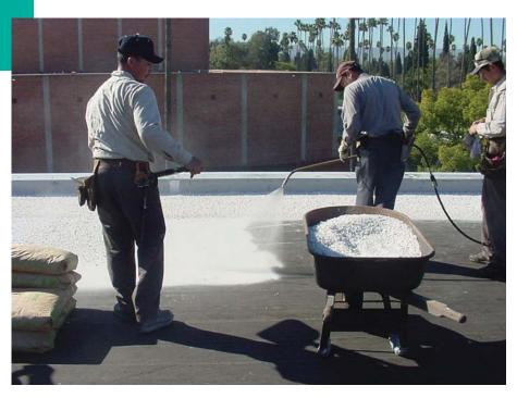
Tremco continues its tradition of leadership and innovation in the roofing industry with the new BURmastic Rock-It Roof Surfacing System, the only cold-process gravel surfacing system for built-up and modified bitumen roofs that meets the strict requirements of California Title 24 Energy Efficiency Standards for Residential and Non-Residential Buildings.
