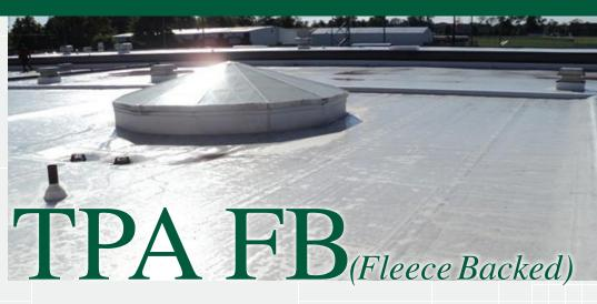
The Tremco Roofing TPA FB system, with its polyester fleece backing, was specially designed for fully-adhered applications. It is particularly cost effective on concrete roof decks and roofs with unusual curves and slopes.
