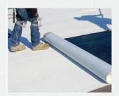
Two options are available to ensure that we can cover virtually any roof, no matter how complex: the white, reflective Tremco Roofing TPA and Tremco Roofing TPA FB (Fleece Backed) membranes. The durable, flexible Tremco Roofing TPA membrane is an excellent choice for roofs that have numerous structures and penetrations. With its polyester fleece backing,
