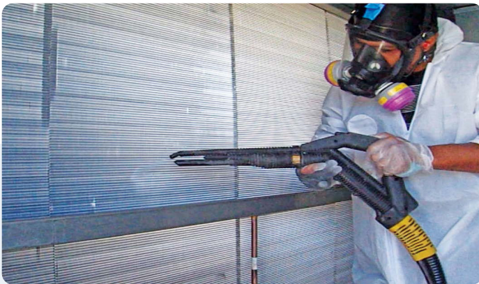
Coils Cleaned
