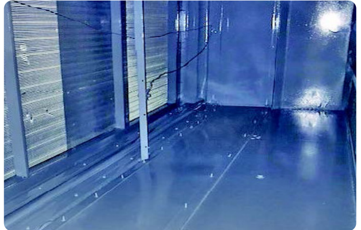
Interior Plenum After Multicoat Siloxane Coating
