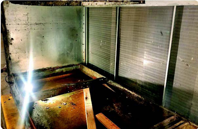
AHU Interior Prep
